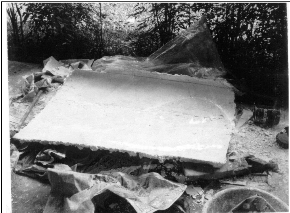
Figure 15: Fiberglass Door Plaster Mold The steel door has just been removed from the mold
